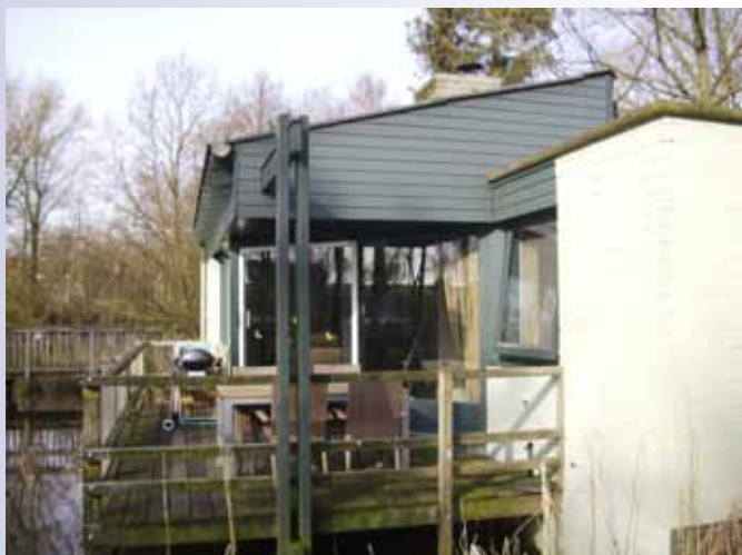
Houtrot reparaties bungalows.
